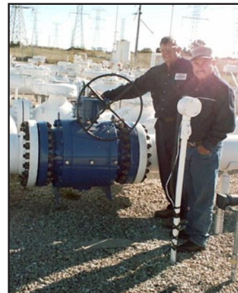
16" DUAL-SEAL BALL VALVE IN UNLEADED GASOLINE SERVICE
