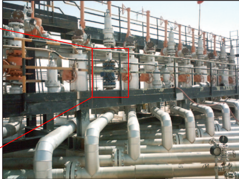
6" 900 WOM Dual-Seal Ball Valve in use in the Middle East
