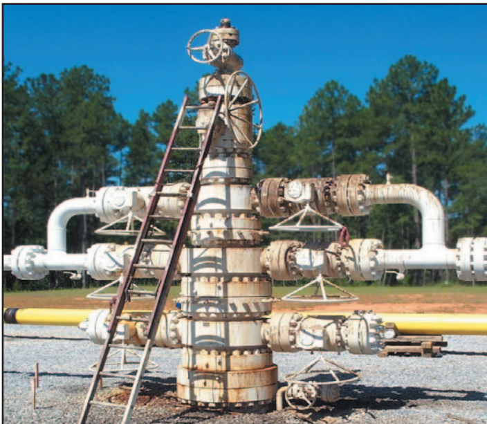
8" 1500 WOM Dual-Seal Ball Valves installed on a natural gas leaching/ storage well in Alabama.
