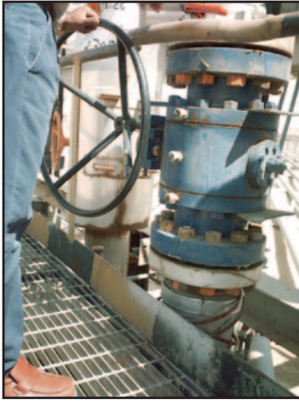
6" 900 WOM Dual-Seal Ball Valve in use in the Middle East
